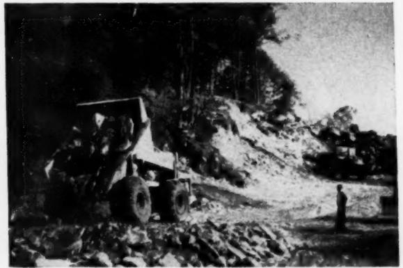
Job No. 2 To relocate Rt. 109 near Watertown, Tournarockers moved 40,000 yds. of rock and 15,000 yds. of gravel on very short hauls (average, 500 ft., one-way). "They're the best hauling units I've seen for limited working areas," says Master Mechanic Phil Onuparik.
